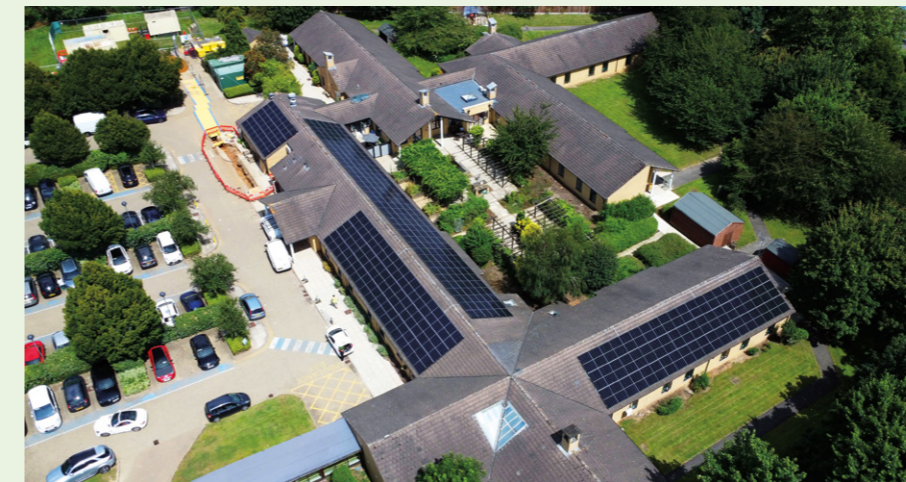
Solar panels on the roof of Langley House Neurological Rehabilitation Unit
